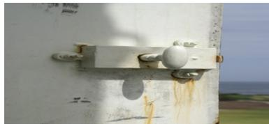
**Note: Historic latch system should be re-used if door is deemed to need to be replaced with new material.**
