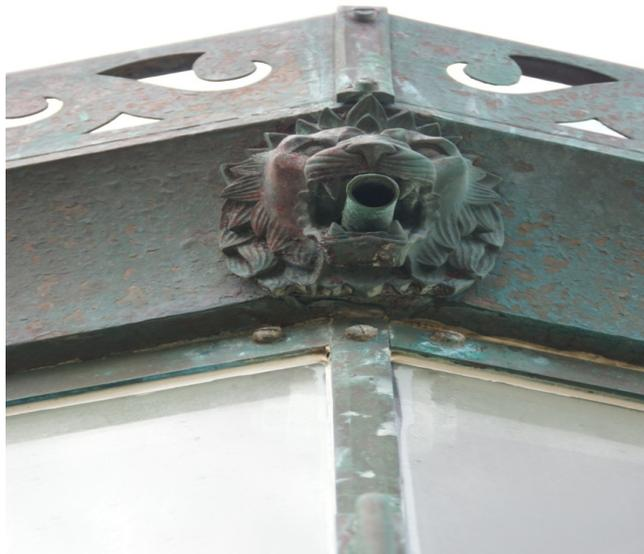
Figure: Bronze Lion Head gutter/downspout
