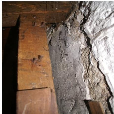
Figure #22: Evidence of earlier plastered wall.
