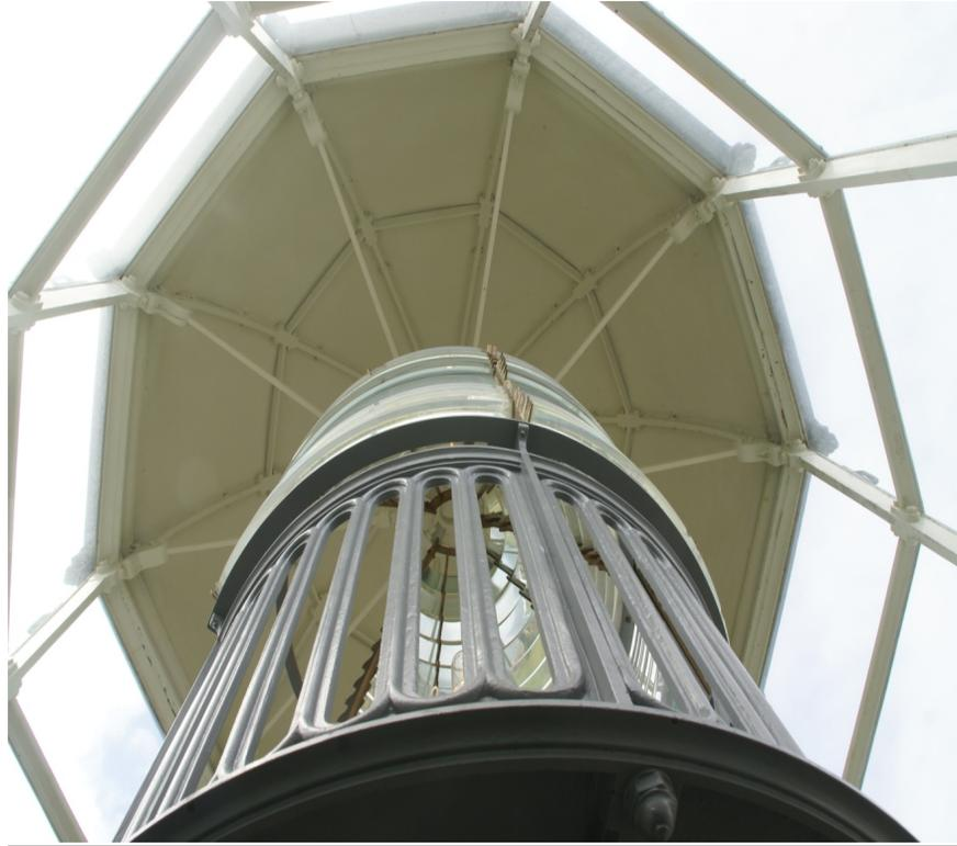
Have contractor perform water test on Lighthouse canopy once it has been re-installed. Have staff member monitor test from inside Lantern Room paying close attention to any moisture penetration into canopy along seam lines.
