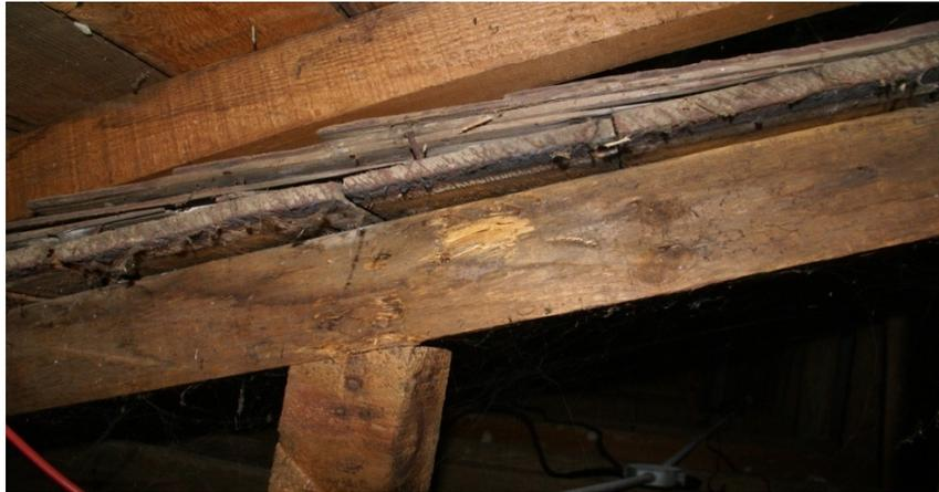
Figure # 21: VIEW OF ATTICI CRAWL SPACE ABOVE ATTACHED KITCHEN AREA. ORIGINAL CEDAR SHAKE SHINGLES FROM PRE-ADDITION WERE STILL IN PLACE.
