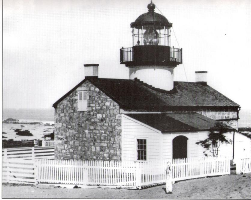
Figure #23: Photograph showing earlier lean to addition to rear-east elevation of Point Pinos Lighthouse.
